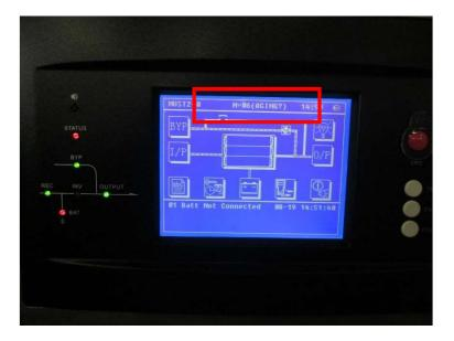
Now you can activate the SefAging, press at same time the bottoms "ENTER" + "ESC". Check that after 1min. the led INV goes ON and on LCD there is written "(A)" blinking.
